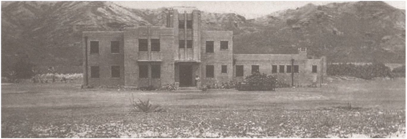
Figure 18. Storm damaged and abandoned Wailua Country Jail in the 1950s (Kaua'i Museum).
